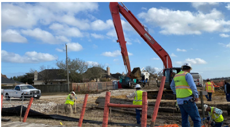
A crew in La Porte working on weld tie-ins.
